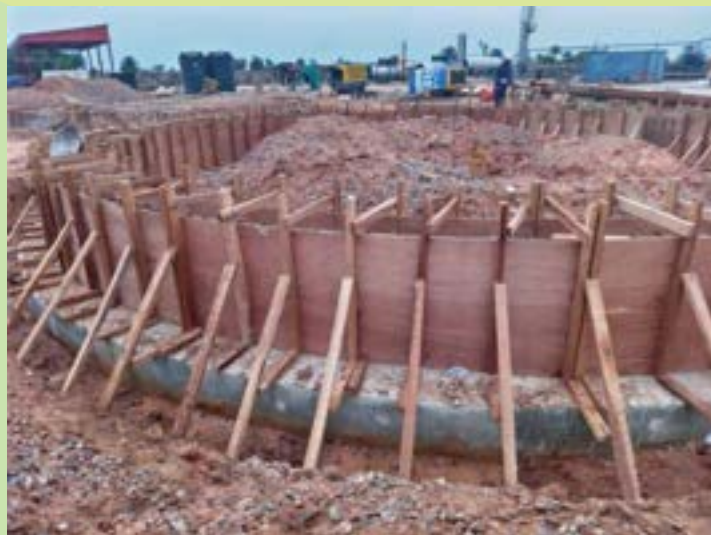
Construction of crude tank foundations
