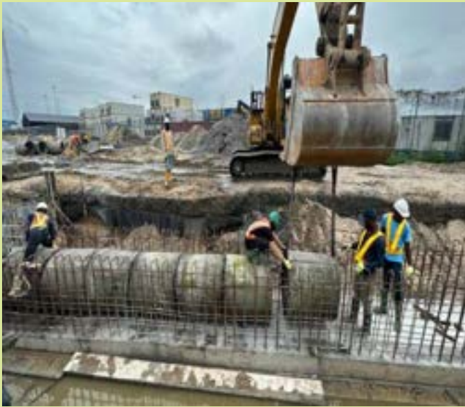
Construction of Drainage Curvet and Company Mac Mixer Truck
