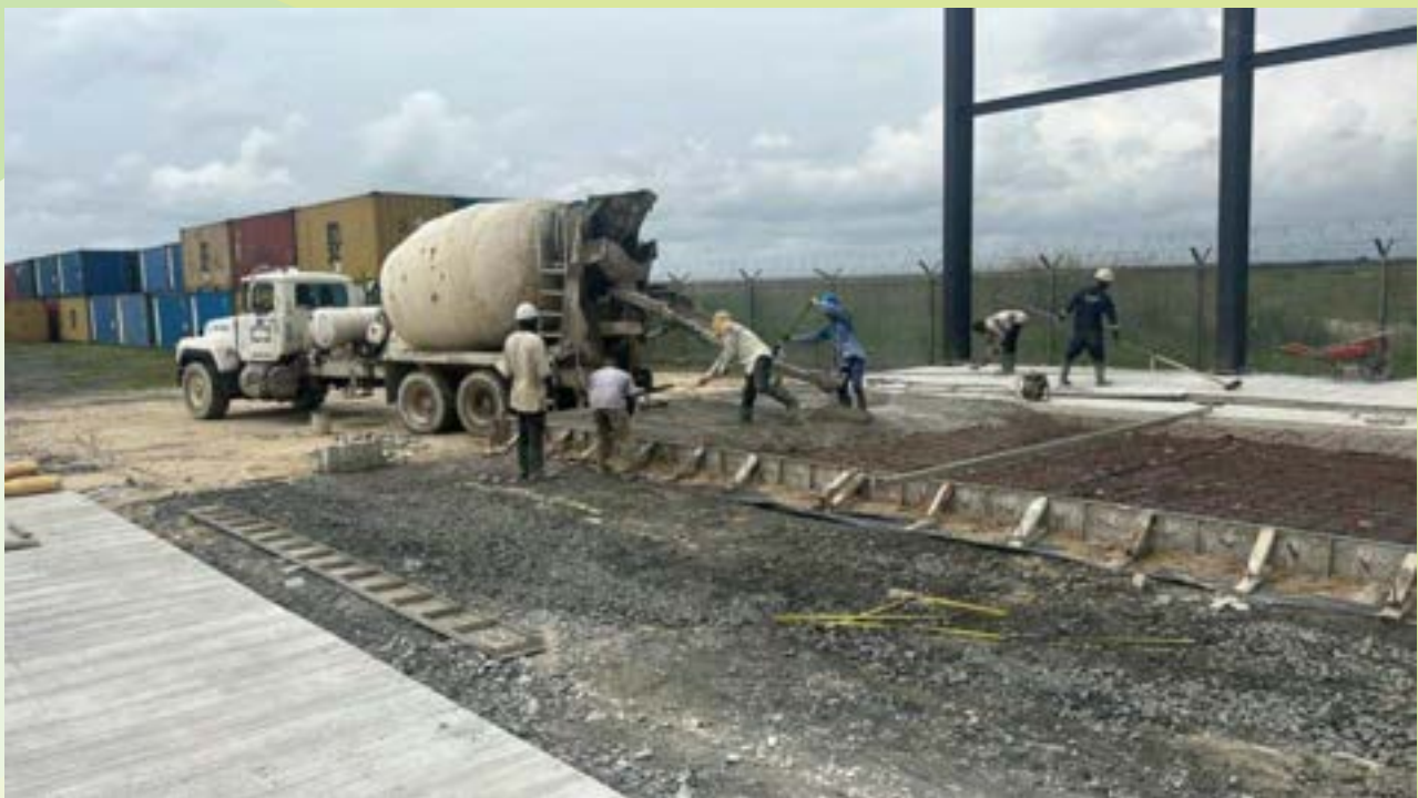
Construction of 30cm Floor paving for warehouse and Drainage Curvet
