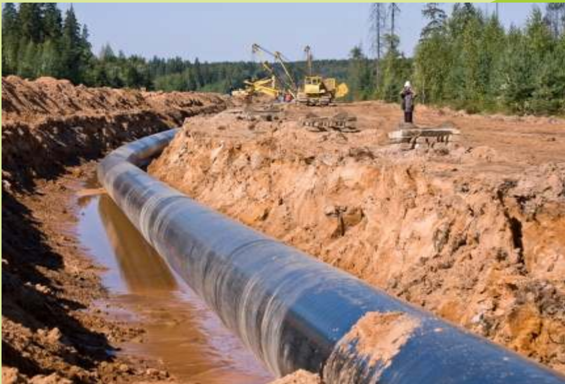
Construction of flow line
