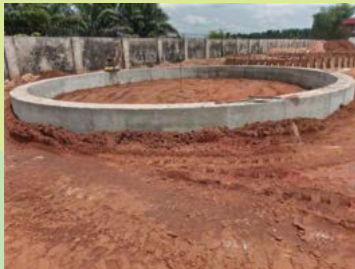
Construction of crude tank foundations
