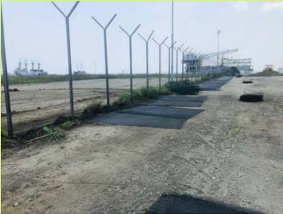
ISPS Mesh Fence Installation 2 and Installation of industrial High Light Mast
