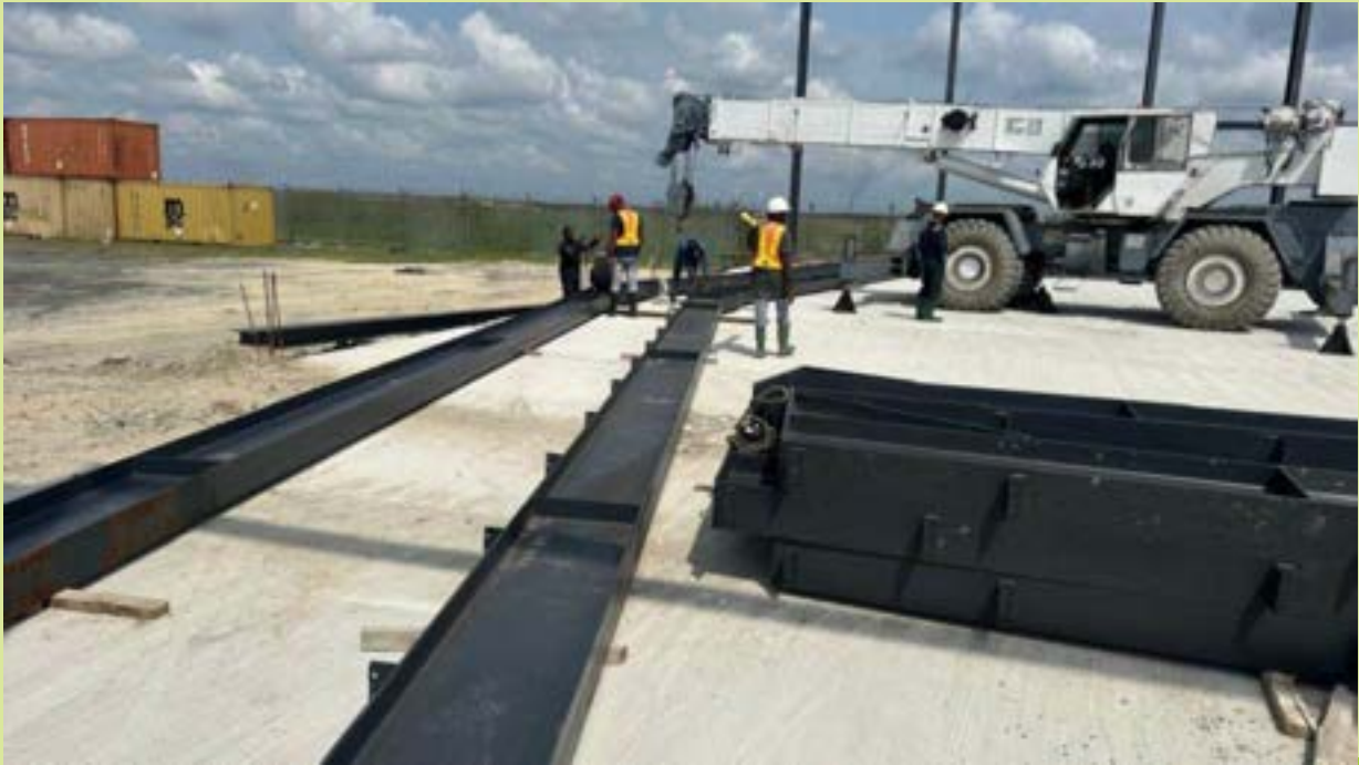
Erection of steel structures for warehouse
