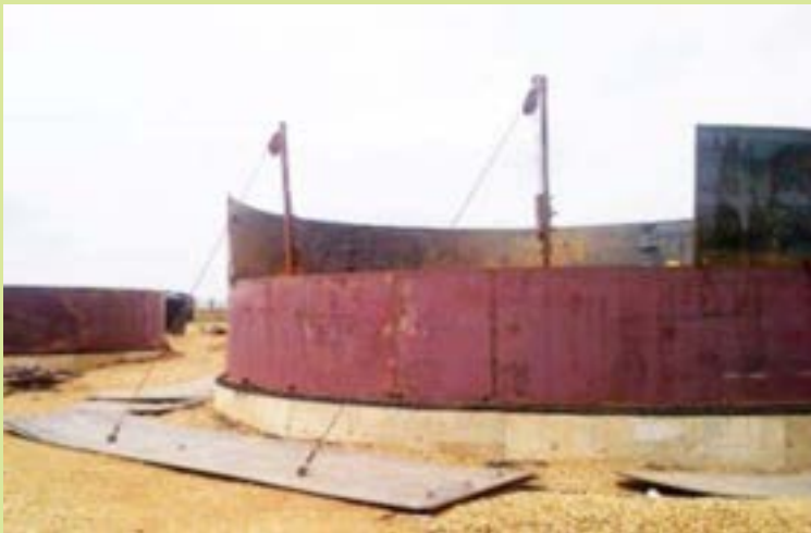
Construction of crude tank
